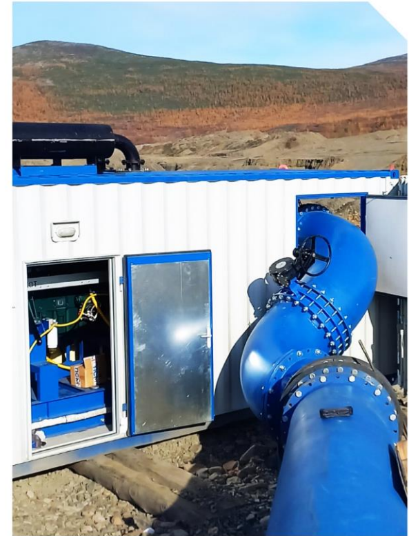
Diesel pump unit for a gold-mining company
