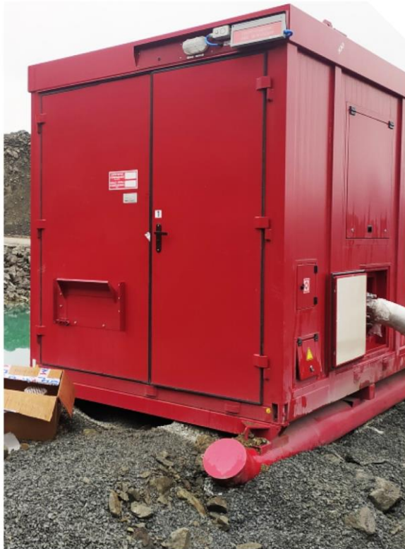
Diesel pump unit for acidic environment pumping
