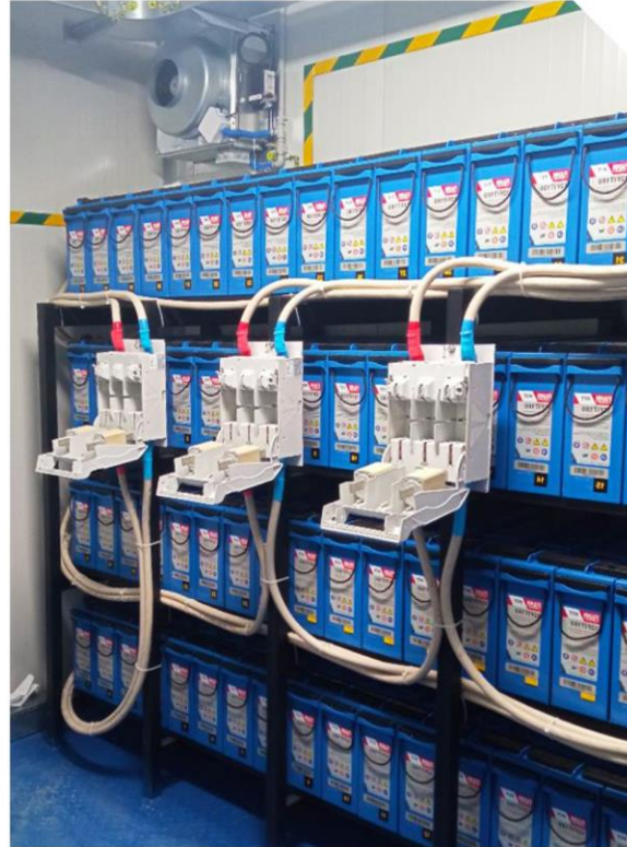
Uninterruptible power supply
