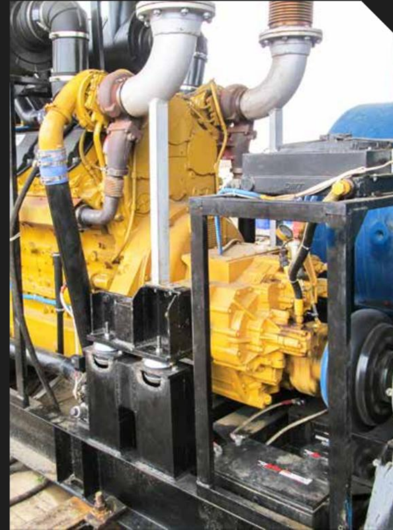
Well drilling pumps
